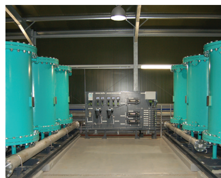
316 m³/h (1400 gpm) Advanced NITRASEP® Plant
